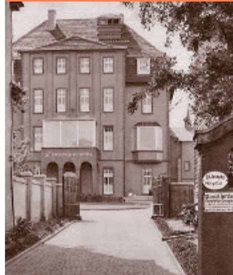
St. Josephs-Krankenhaus, Haan
